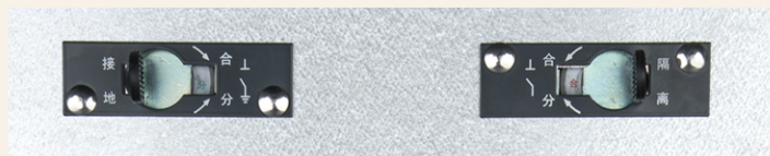
Grounding switch operation
